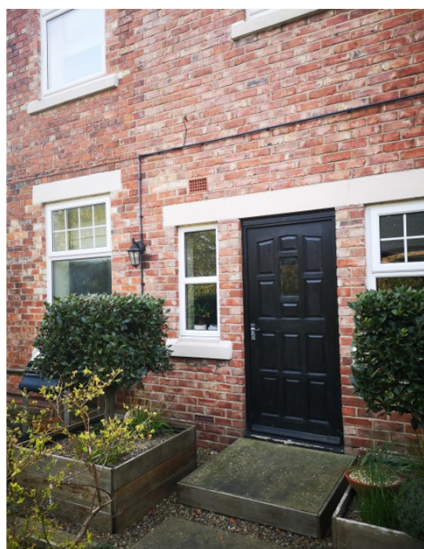
Window, Door and Window to be unified into b-fold doors - East elevation.
